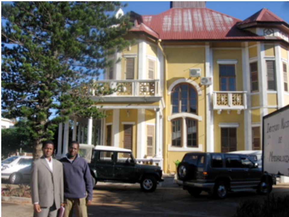
The original, early 20 th century building of the Observatorio Campos Rodrigues, now part of the National Institute of Meteorology (INAM). My hosts Faustino Nhanombe and Claudio Moises Paulo stand in the foreground.
