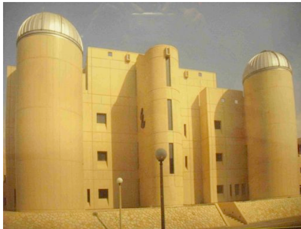
Figure 1 The telescope domes' location at KSU
