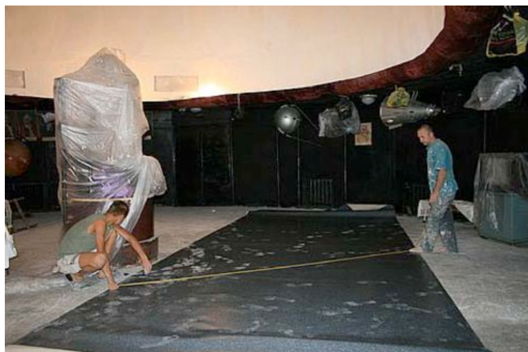
Photo 5, installation of a laser device at the Observatory
